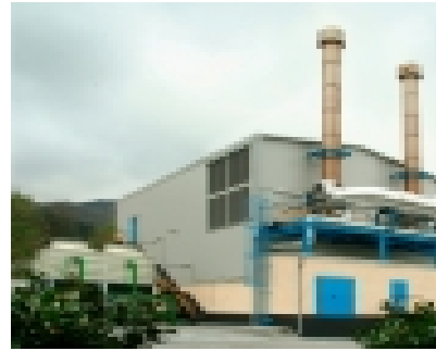
Gas Turbine CHP Plant
